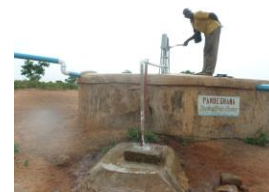
40,000 liters rain water tank
